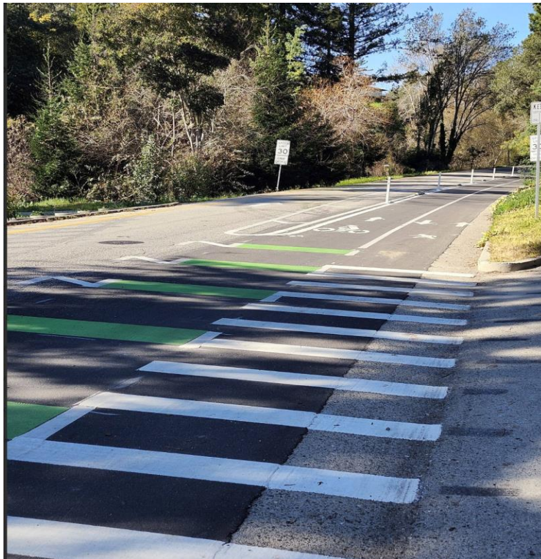
Figure 6- Photo of Bay Ave improvements in the City of Santa Cruz. The road has been narrowed to encourage slower vehicle speeds. Bicycles and pedestrians are separated from vehicles.
